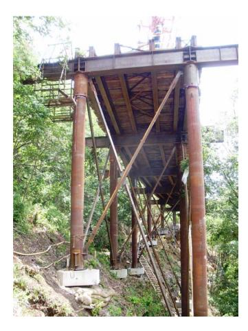
Temporary work bridge to facilitate the top-down construction and erection of a precast balanced cantilever bridge in the Great Smoky Mountain National Park.
